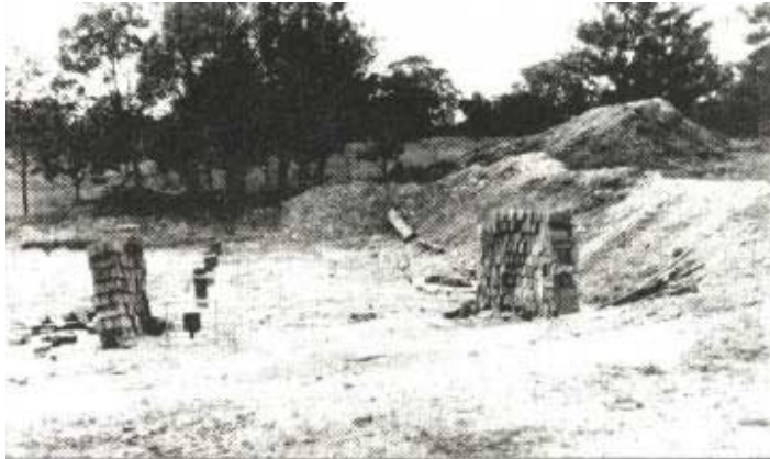
Plate 1 – Earthworks associated with house construction
