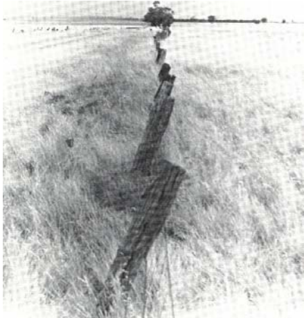
The gilgaied nature of the heavy clays does cause problems with the construction of fences, buildings, roads and other services.
