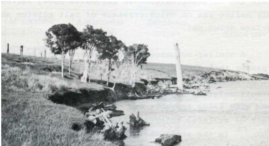
Plate 20 – Erosion on the north shore of Lake King (ECF Bird)
